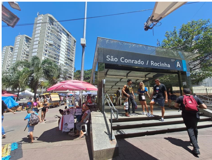
Figure 2 – Entrance A to São Conrado Station
